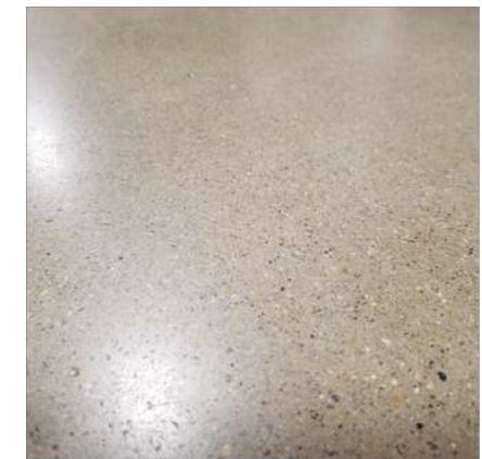
Locker room floors
