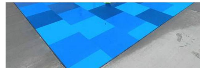
Brushed concrete with inset Lifefloor
